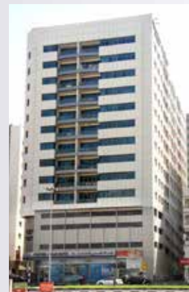
Project: G+3P+10 Floors+Pool & Gym. Location: Abu Shagara, Sharjah Client: Utmost Properties Consultant: Arab & Turk International
