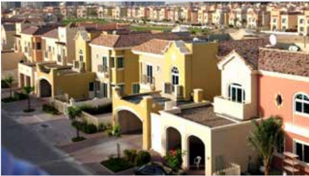
Project: 1000+ Luxury Villas Location: Sports City, Dubai Client: Victory Heights Property Consultant: Diar
